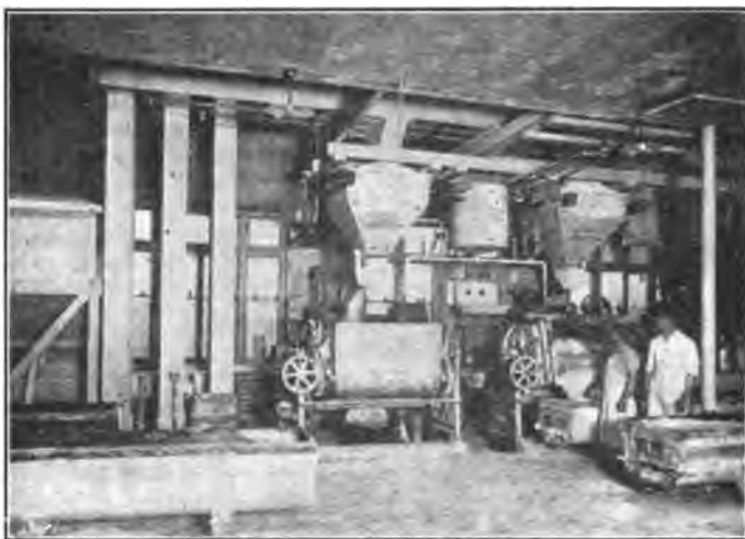
FIG. 12.—Bread mixing room equipped with automatic scales for flour and water as seen above mixers. Brunner Baking Co., Buffalo, N. Y.
